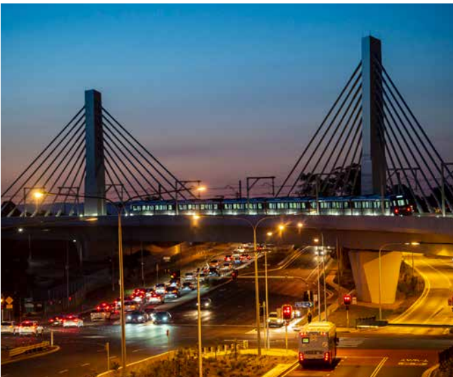
Sydney Metro Northwest. Photograph courtesy of Sydney Metro.
