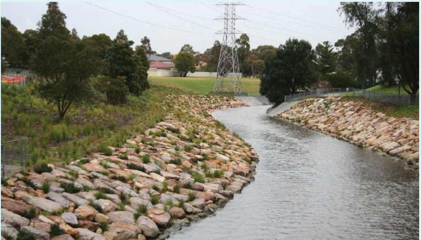
Waterway Naturalisation and Stormwater Improvement, Cooks River.
