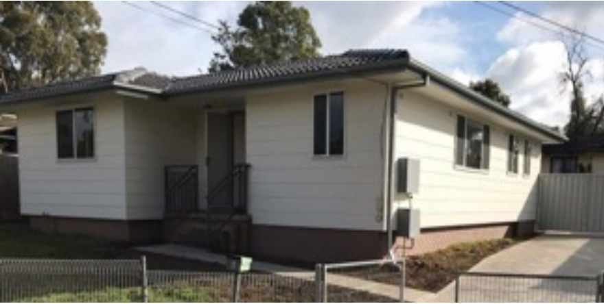
An upgraded social housing property at Windale, Central Coast, delivered by LAHC
