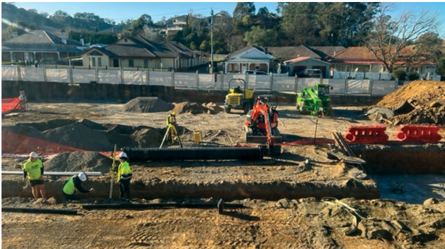
Construction of Wollondilly Cultural Precinct
